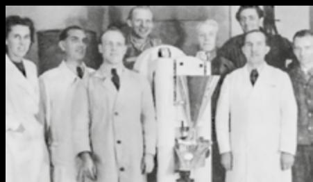
**1948** Fette Compacting presents the first tableting machine developed in-house under the name Hanseaten Perfecta. The press had twelve stamping stations and was able to produce 30,000 tablets per hour.
